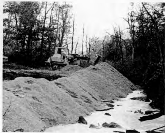
The alkaline sand is placed in windrows along the stream. The current washes the material downstream to neutralize acidity.
